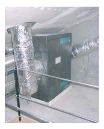
Figure 21: Ventilation unit with heat exchanger in the building services floor of a Hannover-Kronsberg Passive House. In the background is the fresh air duct with defrost heater and in the foreground is the exhaust air pipe (both insulated with mineral wool, aluminium laminated)
