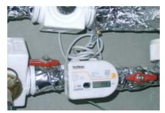
Figure 42: Total heat quantity meter on the installation wall of the building services floor. The cable leads to the temperature sensor (Pt 500) in the supply pipe.
