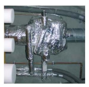
Figure 22: Postheater in the inflow pipeline (before and after the addition of insulation)
